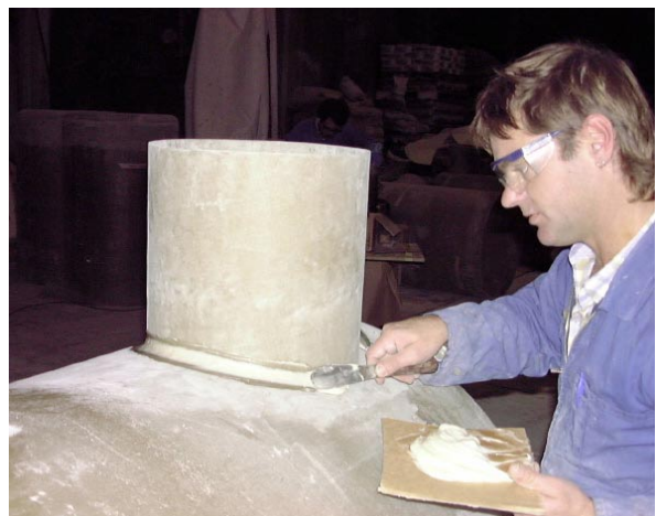
Armabond VE putty being used to fit and join a fibreglass pipe stub to a fibreglass vessel.
