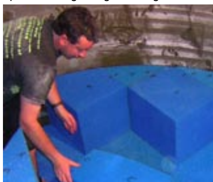
Inorganic packing being installed by ARMATEC.
