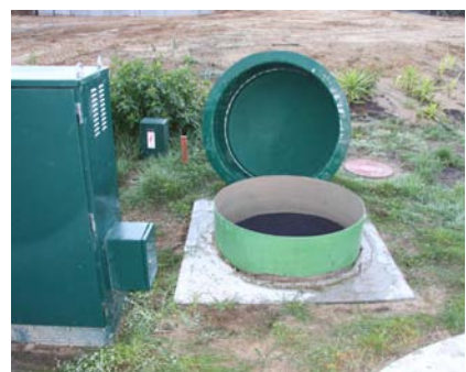
Place carbon in unit and level. Note the top of the base module must be well above any possible local water level.
