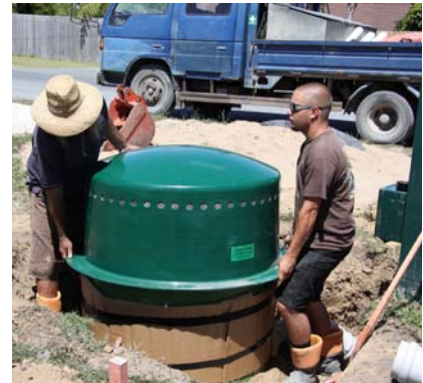
Place base module in place, connect duct and check final height of top module.
