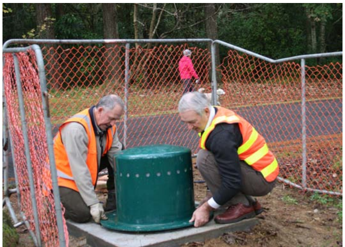
Left: Carbon loaded into base module, with room for more carbon if needed. Top of base module above ground, so carbon cannot be flooded by ground water. Right: Top module bolted back in place.
