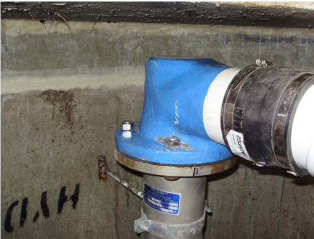
Left: Flanged fibreglass low profile fitting to match air release valve. Flexible joint allows for thermal expansion and contraction. Right: Green Dome base in concrete pad to secure in position.
