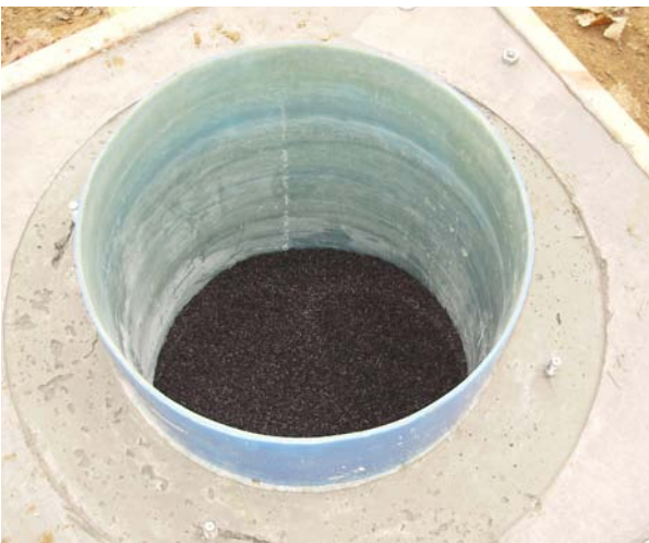
Left: Carbon loaded into base module, with room for more carbon if needed. Top of base module above ground, so carbon cannot be flooded by ground water. Right: Top module bolted back in place.
