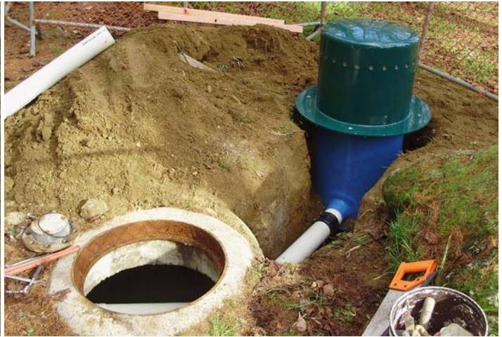
Left: Same hole through concrete manhole used for duct to Green Dome. Right: Duct sloped towards Green Dome to drain condensation away through holes in base module. Heights set to suit local ground levels.
