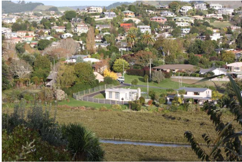
Photo 2: Otumanga Pump Station, Welcome Bay, Tauranga
