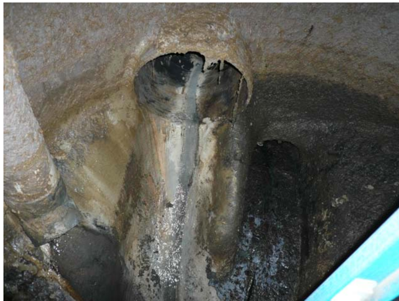
Photograph 4: Base of deep manhole in municipal sewer system coated with moisture tolerant and chemically resistant ARMALINE 1730 epoxy coating. Again, complex shapes require rehabilitation by coating.
