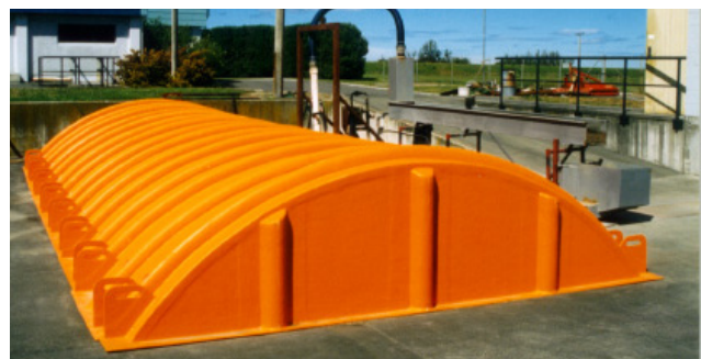
Fibreglass cover over open sewage channels and grit separation tank to contain H 2 S odours.
